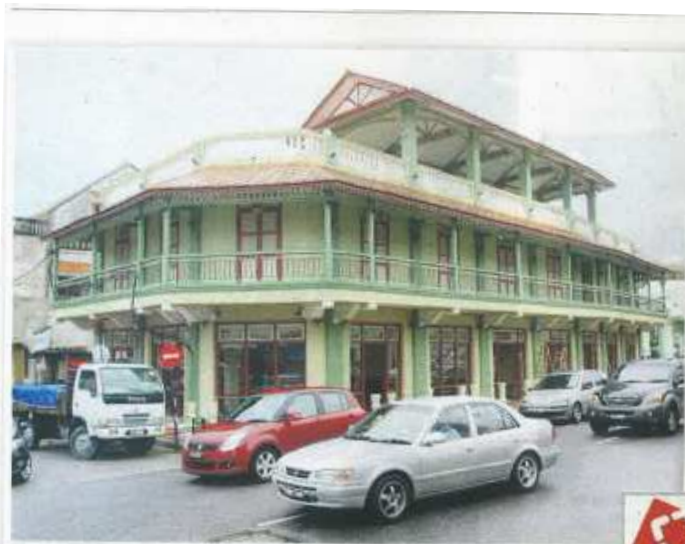
Standing proud: Loke Thye Kee building in Burma Road, George Town.
